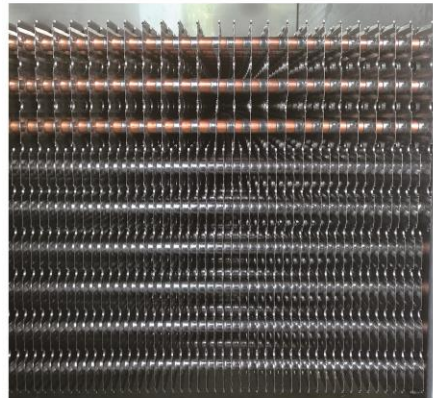
# Dual fin space, front 16mm, back 8mm
